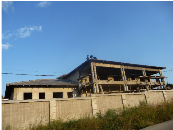
Shell almost finished
