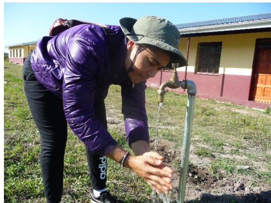
Valencia tests the water from the MEDEA-built borehole
