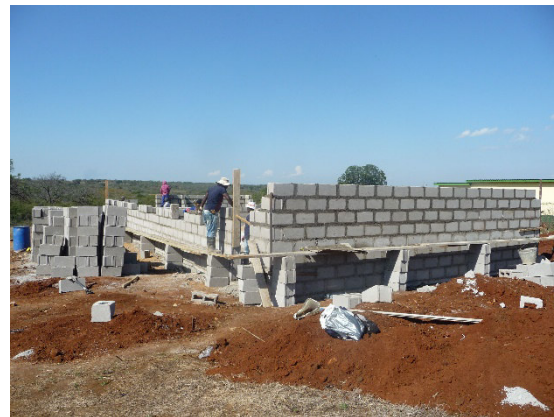
Pre-school building is growing
