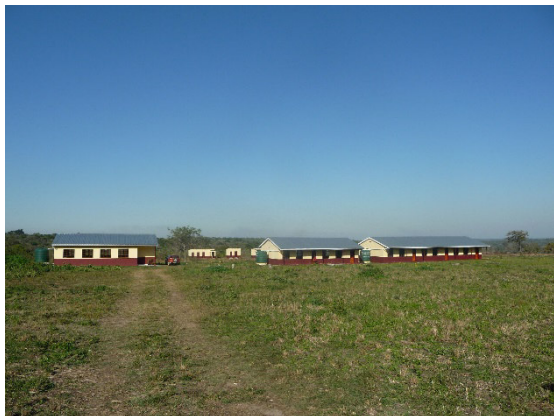
View of High School (left laboratory, right classrooms, in the background sanitary building)
