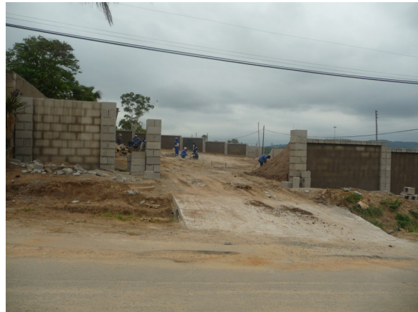
Start of construction, the outer wall stands
