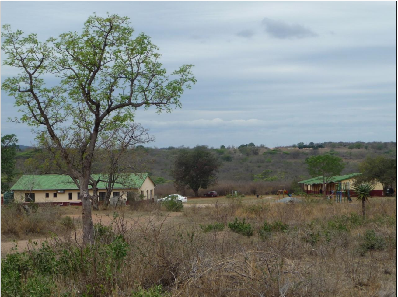
Administration building (left) and classrooms (right)
