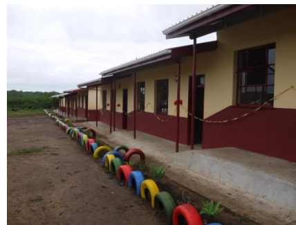
The 3 new classrooms
