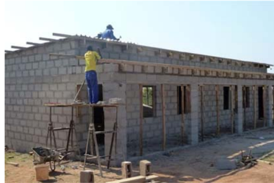
the shell is nearly completed
