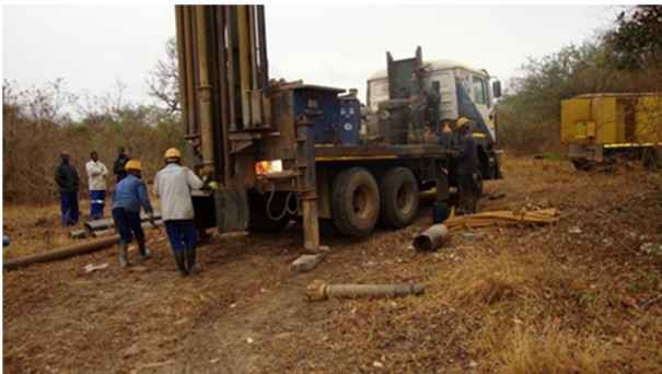
Driving heavy drill machine
