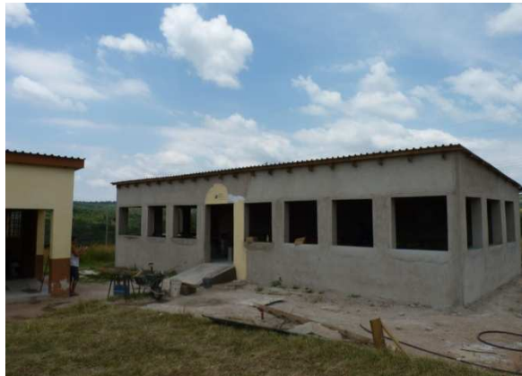
The basic structure is finished.
