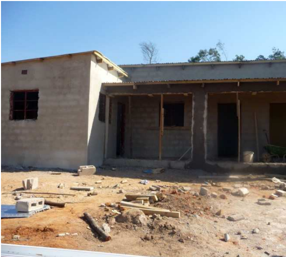
Front view of the new housing
